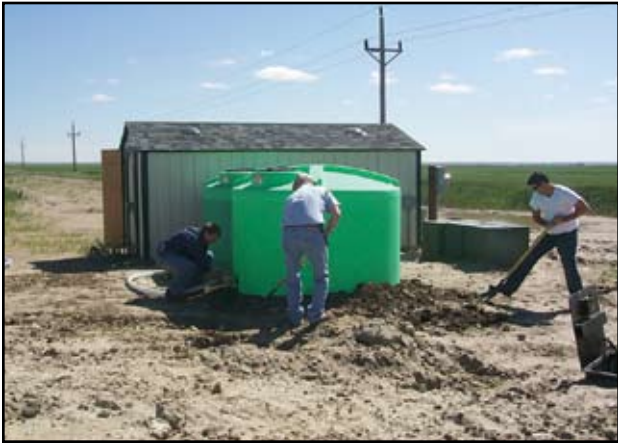
Adding a tank to the free product recovery
